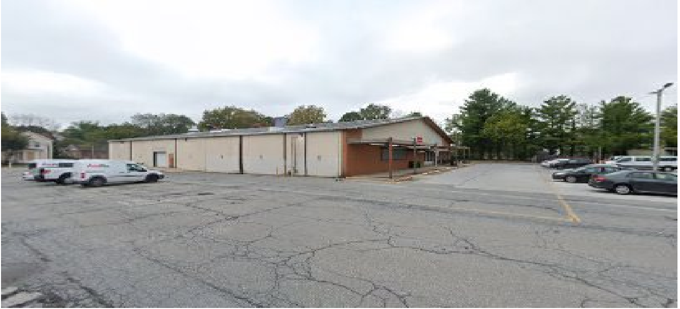
120 South Governor's Ave- Remediated and Demolished
